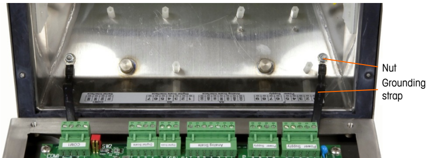
Figure 3-11: Loosening the Ground Straps
