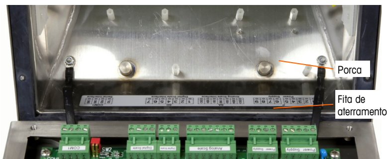
Figura 3-11: Soltar as fitas de aterramento
