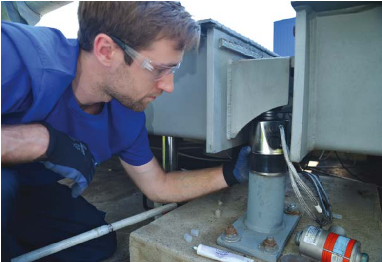
Conversion kits make it easy to upgrade existing vehicle scales POWERCELL® PDX® load cells.
